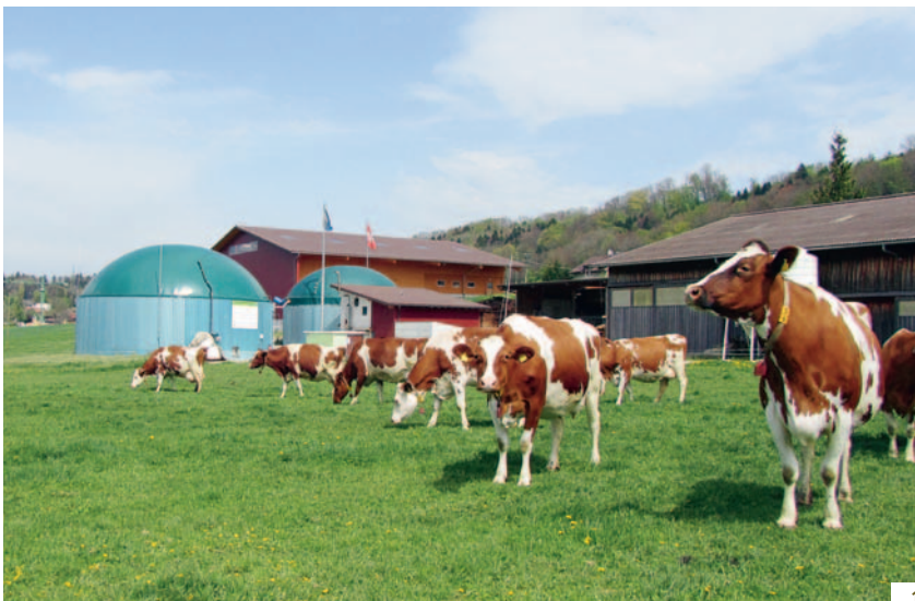
1_ Eco-electricity is generated in biogas plants on Swiss farms – supported and co-financed by Swiss Post.
